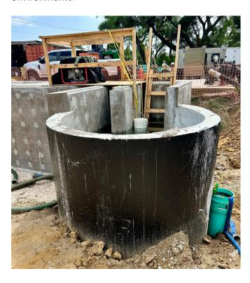
The influent channel and grit cell infill were treated with Xypex Bio-San, providing protection against microbial-induced corrosion (MIC), significantly reducing maintenance needs, and extending the infrastructure's service life.
